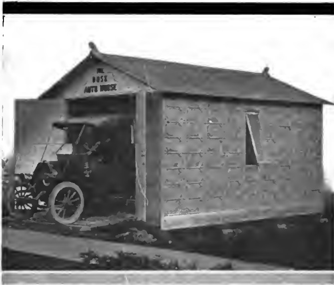
Fig. 3—Fireproof Rusk garage of gable type with ornamental pressed steel sides and hinged window
